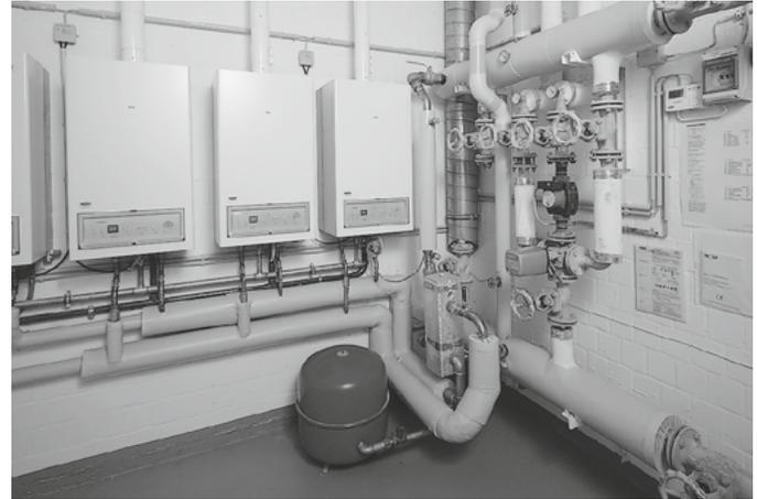
*Each heating boiler in a cascade is controlled by a dedicated heating controller.*
