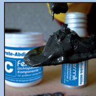
4. Pre-shape a setting filling plug of sufficient size on the spatula.
