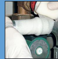
2. Pipe is unpressurised and cold. Place of repairs is clean and moist. Wrap round bandage quickly and tightly. (thickness 6 mm).
