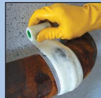
8. Finally swathe with the fermit sealing bandage as described.
