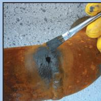
3. Apply a basic layer around the place of repair.
