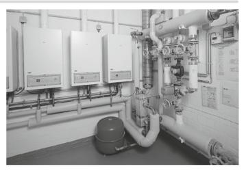
Each heating boiler in a cascade is controlled by a dedicated heating controller.
