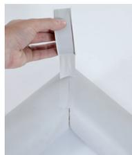
Seal the longitudinal seam with the self-adhesive overlap and the butt joints with suitable adhesive tape.
