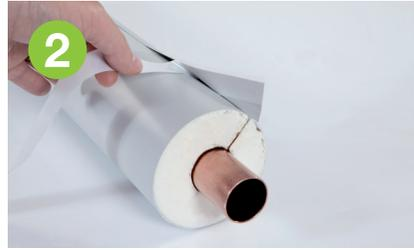
Press the longitudinal joint together, peel off the protective strip of the closure and press the adhesive tape down firmly. **The surfaces to be bonded must be dry and free of dust or grease.**
