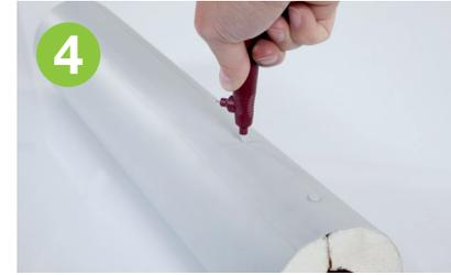
Alternatively, the overlap of the longitudinal seam should be fastened with rivets. At ambient temperatures above +40 °C and on pipes which will not be accessible later, the seam should be additionally secured with plastic rivets (at least 5 per metre).
