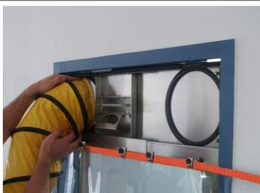
Now – depending on the use (see Section 5) – one or two hoses (Ø 203 mm) can be drawn through the openings of the DCD.
